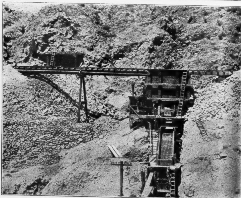
Top—The Storage and Dock. Bottom—The Trestle Bins and Crusher Feed
